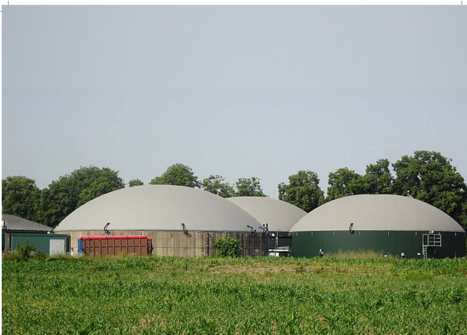
Barsana Biogas Plant, Mathura, Uttar Pradesh- India's largest agri-waste-based bio-CNG facility
