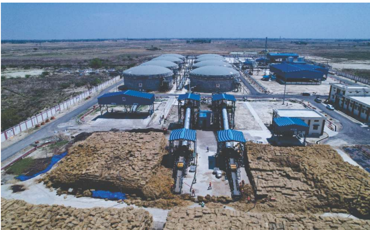
Fig 4: 200 TPD paddy straw based CBG in Gorakhpur, Uttar Pradesh
