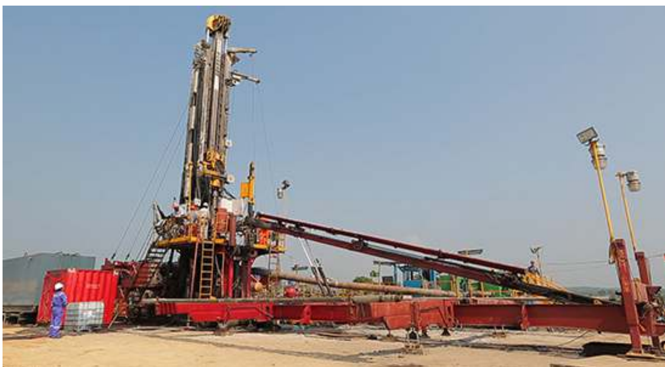
Raniganj CBM (Coal Bed Methane) Facility in Burdawan district of West Bengal
