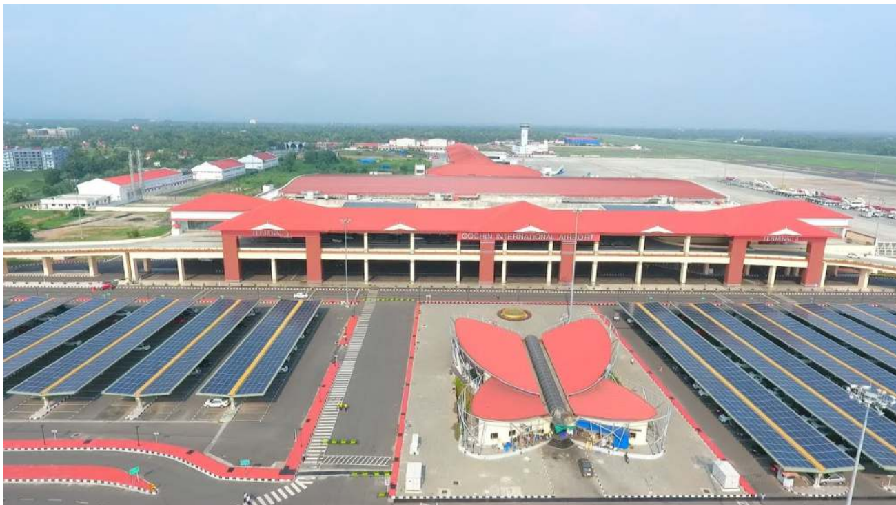
Cochin International Airport- World's First Solar Powered Airport
